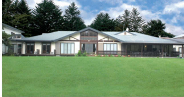
Training course facilities and accommodation facilities Karuizawa YUAI Cottage
